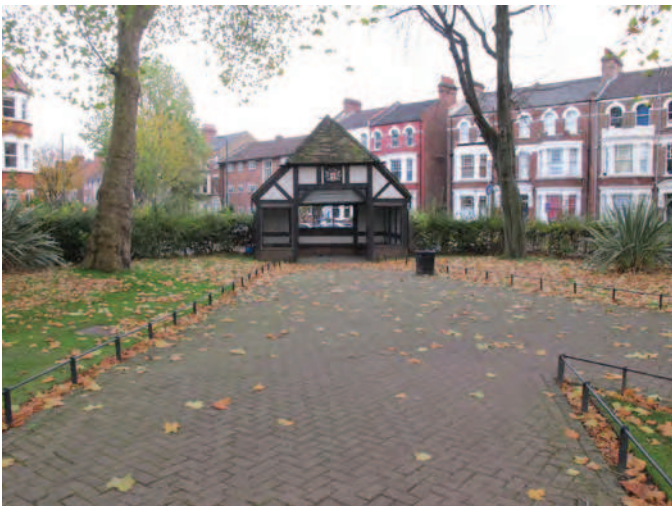
View south towards Lych Gate
