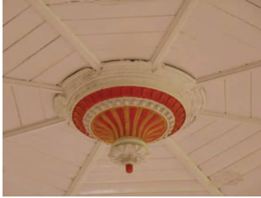
Detail of ceiling
