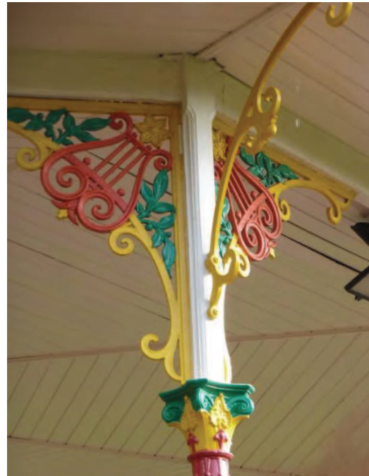
Detail of column bracketry
