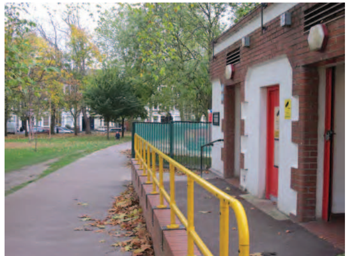
View south of toilet block
